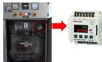
Fig. 4: The installation of Eco Power Meter to measure the amount of the electrical power used
